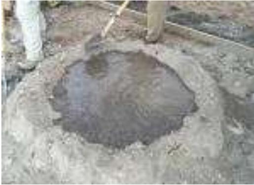
Fig. 2. Mixing of concrete
